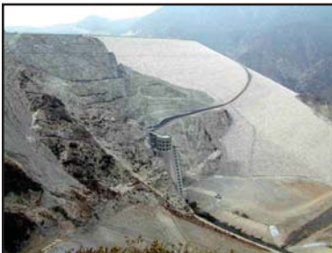
Seven Oaks Dam Source: Army Corps of Engineers Website
