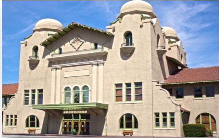
Metrolink's San Bernardino Depot Station, located in the City of San Bernardino. Photo Courtesy of Metrolink
