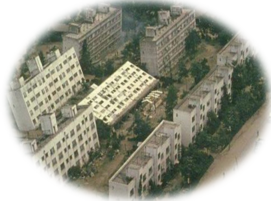
Liquefaction caused by the 1964 Niigita, Japan earthquake caused these apartment blocks to experience severe leaning. Image from the University of Washington.
