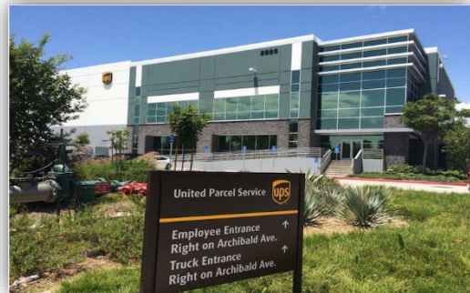
UPS air and ground sorting facility at San Bernardino International Airport. Image from Connectcre.com
