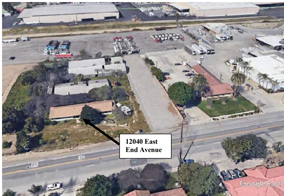
Figure 2: 3D Aerial view of 12040 East End Avenue w/ outbuildings, March 2017.
