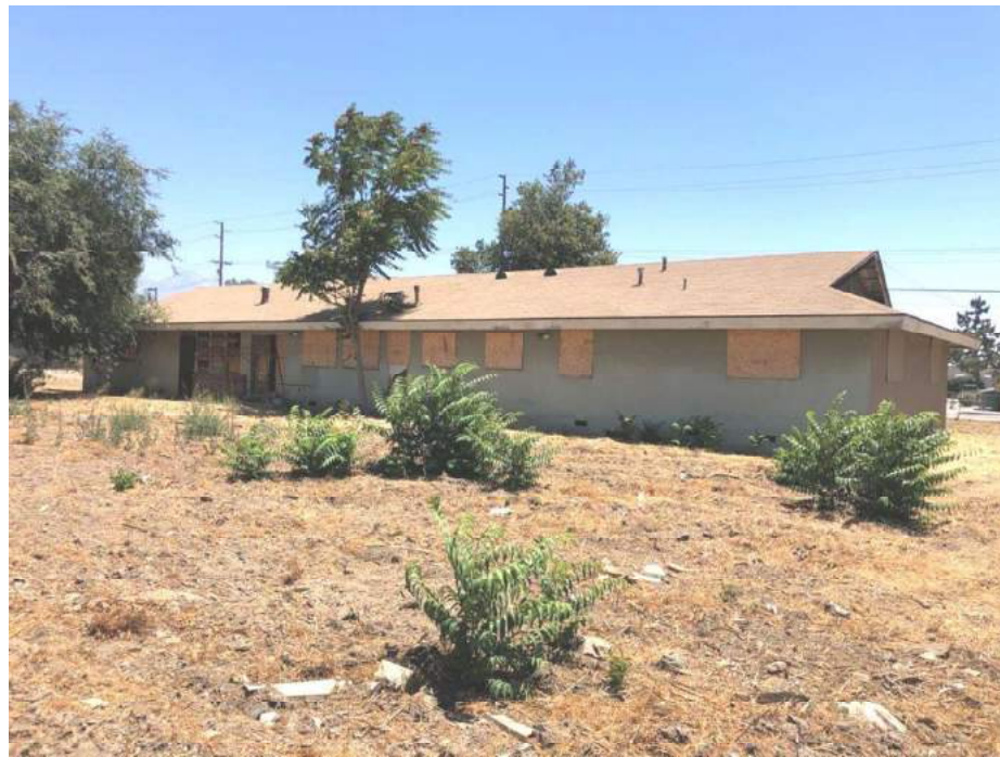
Photograph 2: View looking southeast at the rear of the residence.
