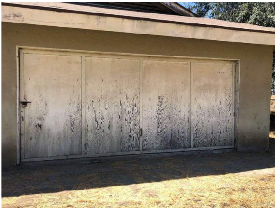
Photograph 8: Close-up of the east elevation garage door.
