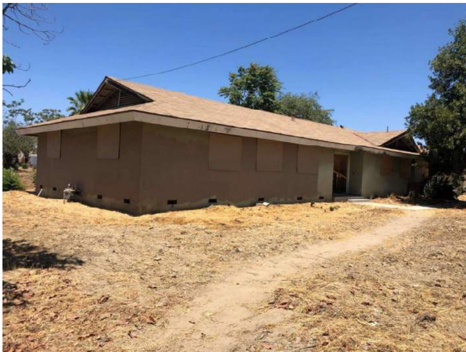
Photograph 4: View looking northwest at the front of the residence.
