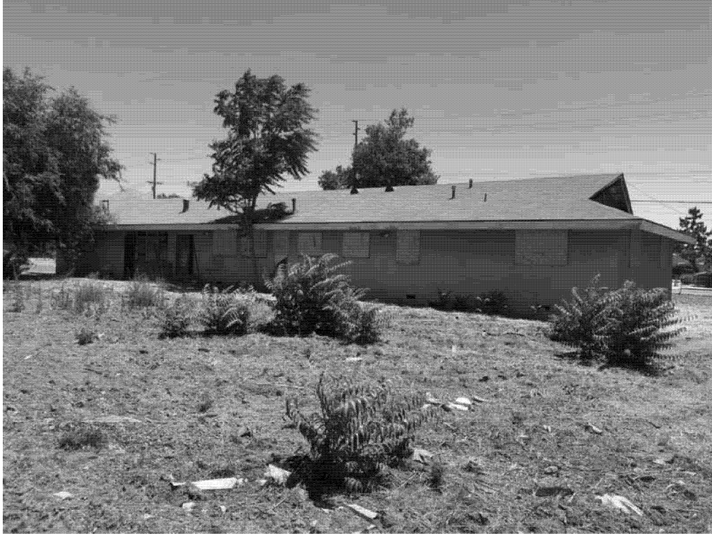
Figure 5: Overview of house, view north.
