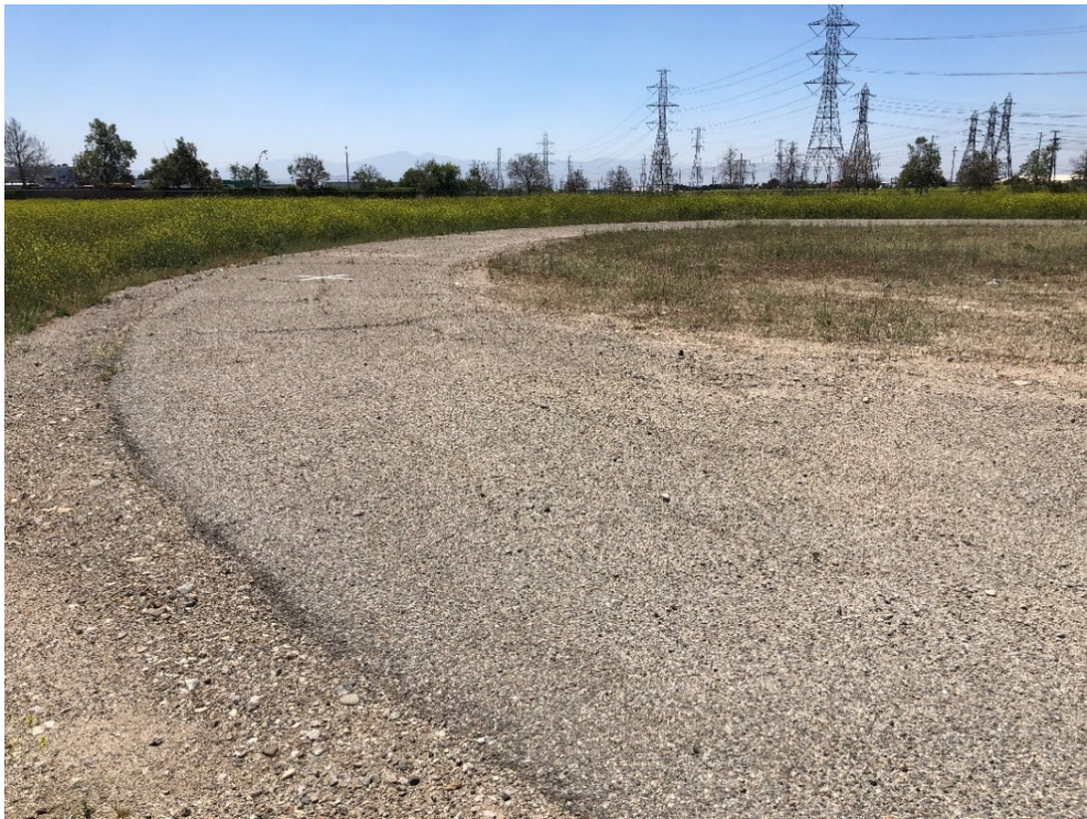
Figure 5-4 View of asphalt road, view to the southeast
