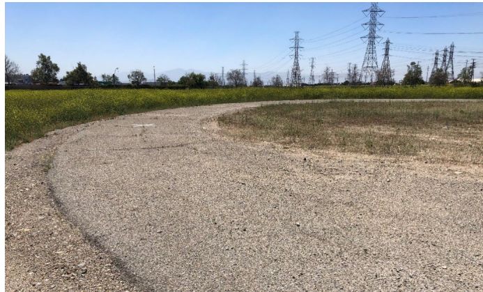
View of asphalt road remnant, view to the southeast
