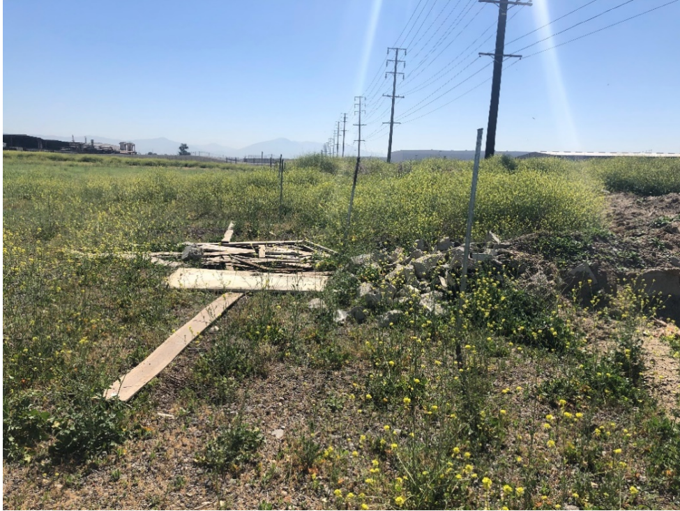
Figure 5-3 View of concrete and wood debris and transmission line, view to the west
