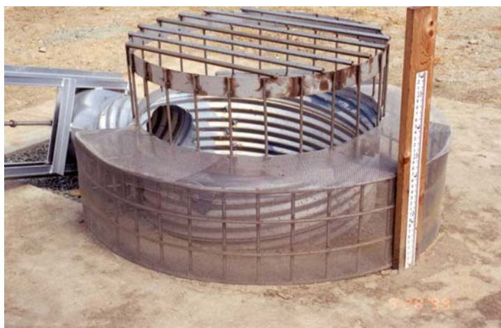
Figure 1 Example of Extended Detention Outlet Structure
