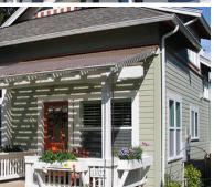
By taking into account solar orientation of the building, overhangs and other devices placed on the exterior of buildings reduce direct sunlight into interiors, lowering heat gain and the amount of energy needed for cooling.
