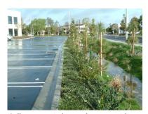
Collect water in bioswales to provide a cost-effective alternative to traditional stormwater drainage systems and serve as landscaping buffers.
