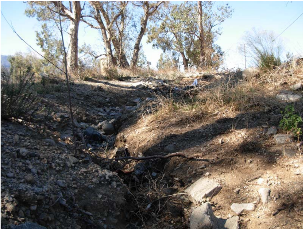
Photo 10: Looking Upstream Tributary 1A
