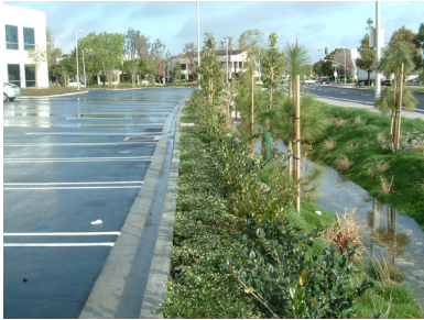
Collect water in bioswales to provide a cost-effective alternative to traditional stormwater drainage systems and serve as landscaping buffers.
