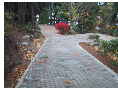
Permeable paving materials allow water and air to filter through to the ground underneath, reducing stormwater runoff and associated need for standard drainage infrastructure.
