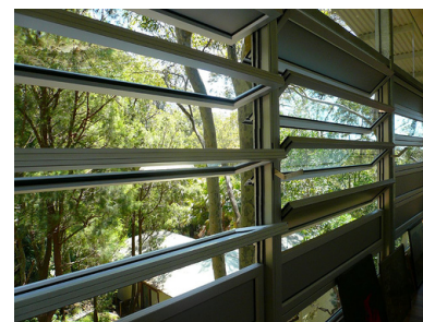
Operable windows allow natural air flow through interiors, reducing energy needed for cooling.
